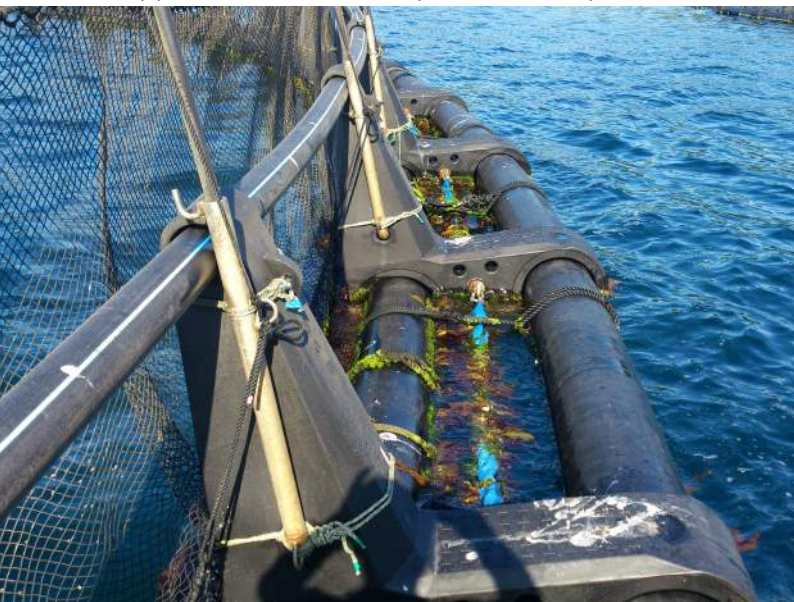
Pole support tied to handrail uprights with ropes.
