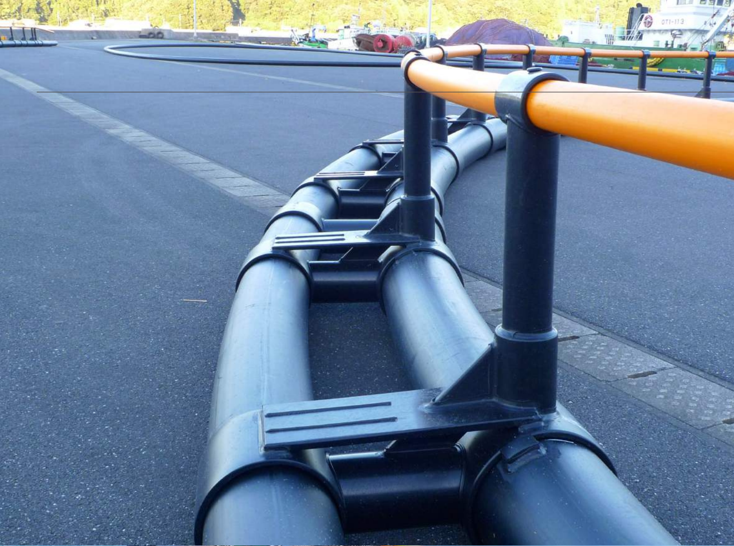
35m-diameter cage with balanced stanchions, 355 & 315mm floating pipes. Oita, Kyushu, Japan
